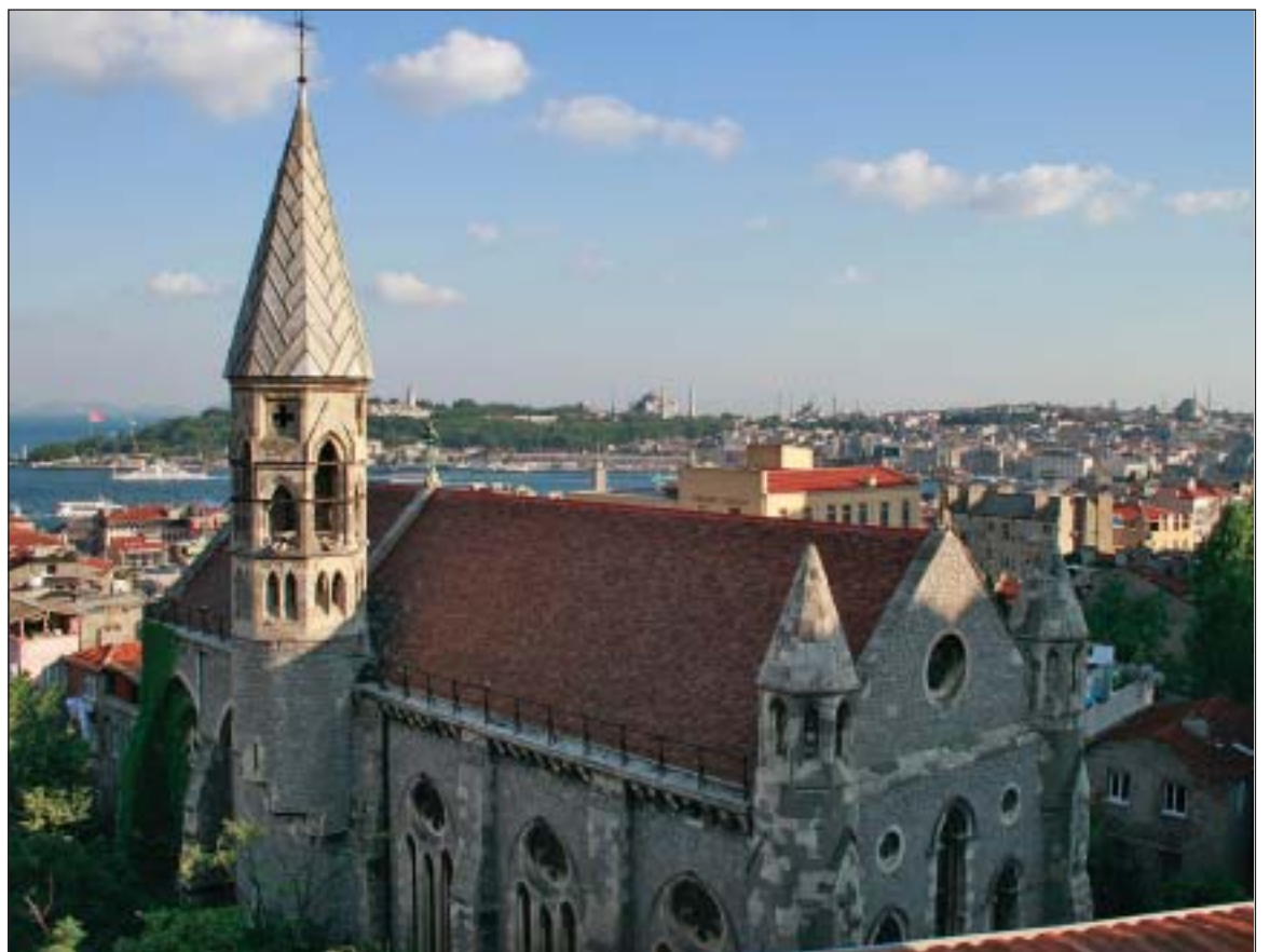
Looking south over the roof of Christ Church, towards the heart of Istanbul. Photos by the Rev. W. Tay Moss
